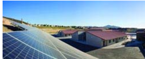
Monterey Ridge Elementary School is Poway Unified School District's first solar-powered school.
